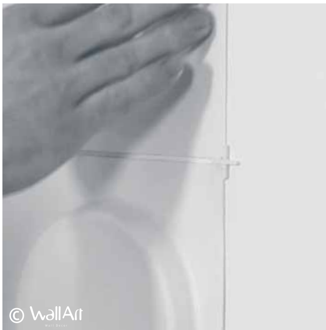
Install Wall Panel using Tile Spacers (different size available)
