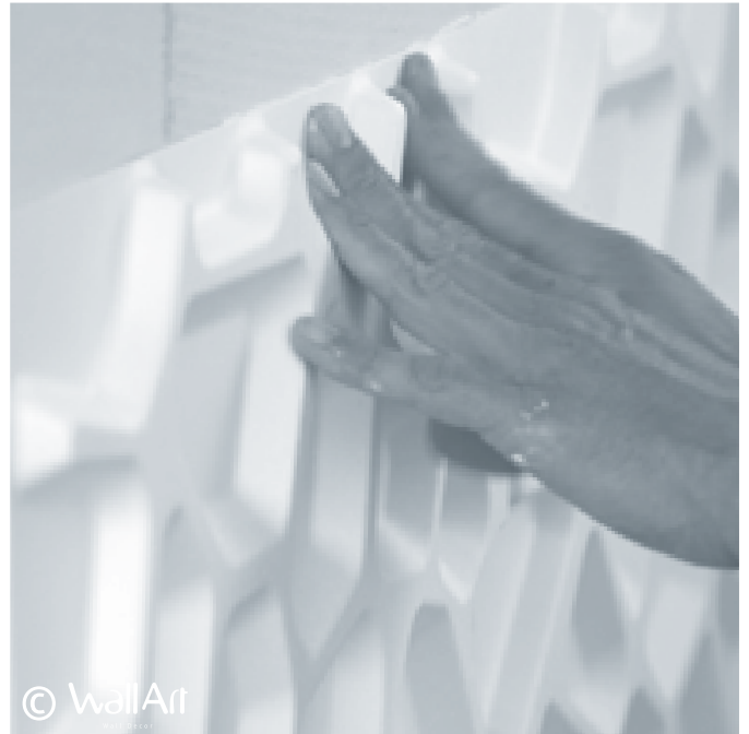
Install the cut to size panel on the leftover space.
