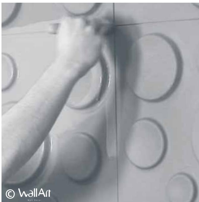
Second layer of paint
