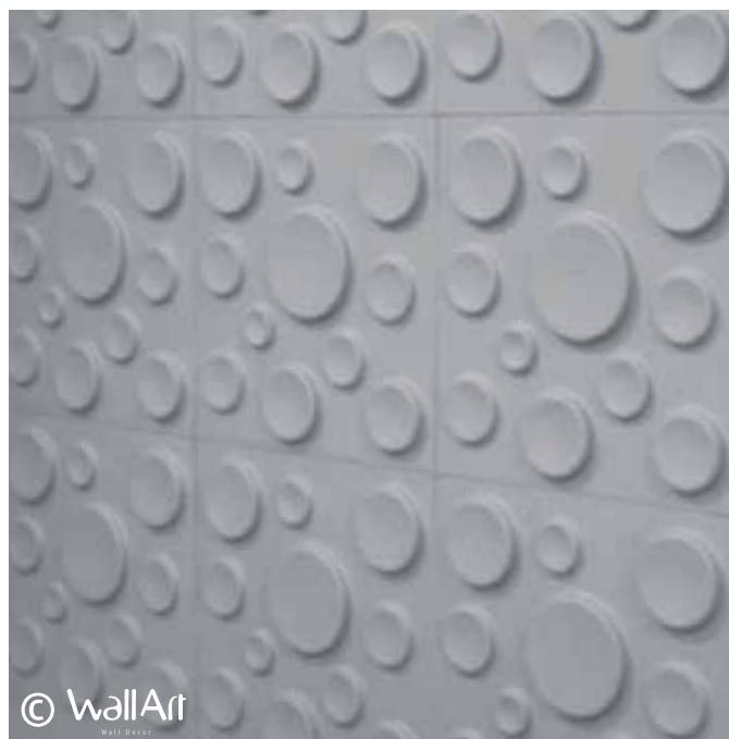
Result of Wall Panel installation without filling the Joint seams
